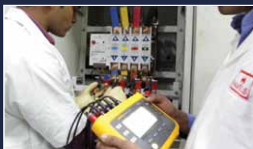
LOAD FLOW & HARMONICS ANALYSIS
